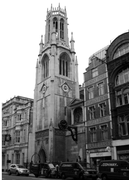
St Dunstan in the West with the former Dundee Courier building next door.
