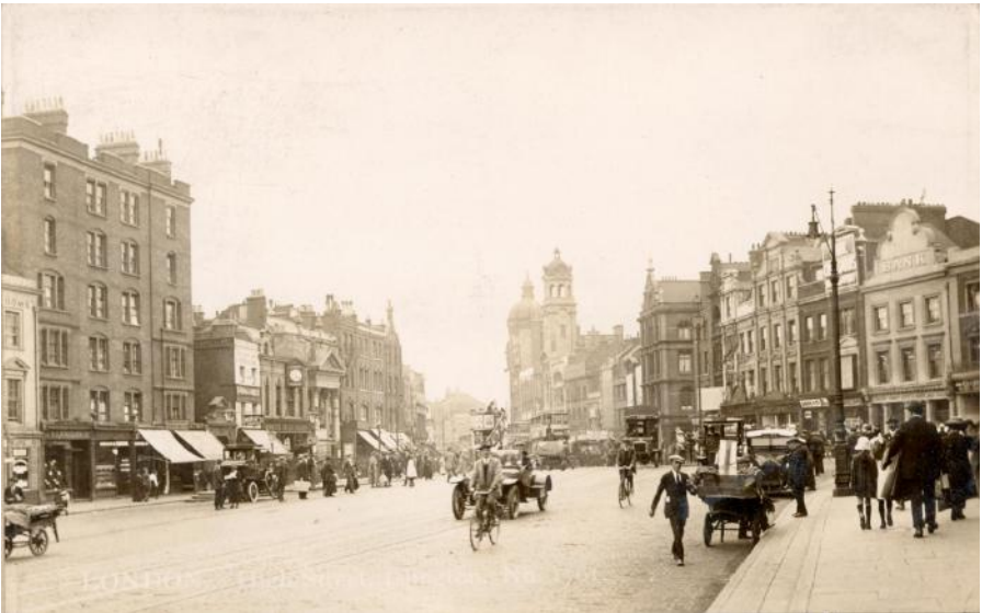
Islington High Street looking towards the Angel, 1920s
