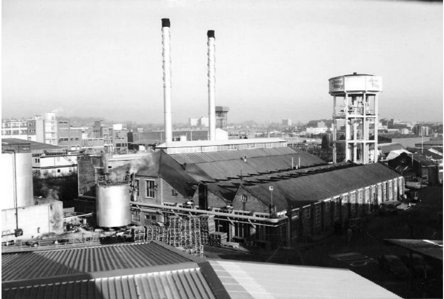
Photograph of the Greenford site taken from the Tea Factory showing the Boiler House. In the left background is the Ice Cream Factory, Bridge Park. The right background shows the Glaxo Factory.
