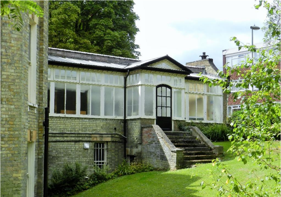
The unusual covered walkway from Lyonsdown Road to the main part of the house
