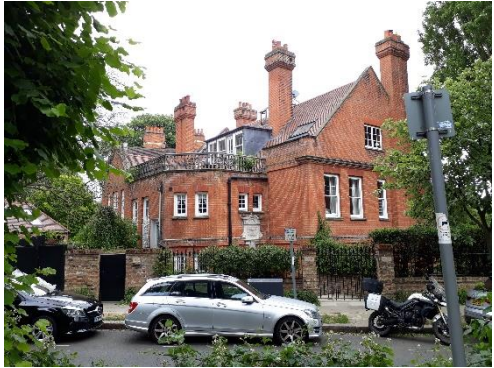
The former Pump House in Well Walk.
