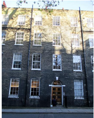
Charles Dickens worked as a clerk for Ellis and Blackmore, who were based at Raymond's Buildings here in the 1840s.
