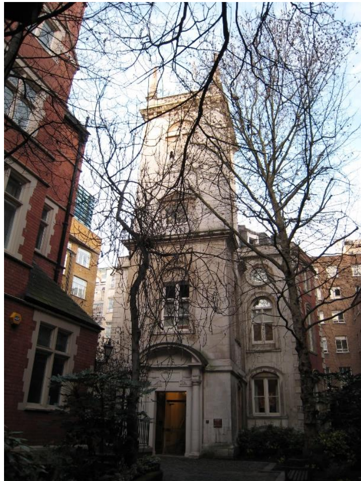
The tower of St Olave – now an office building
