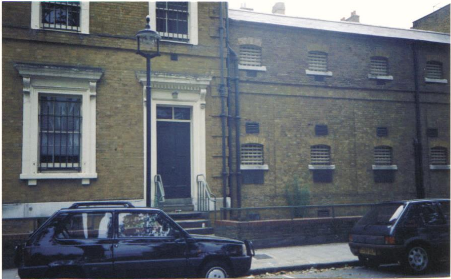
The Vincent Square Police Station, showing the cells on the right.
